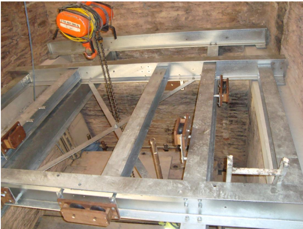
New foundation girders for the bell frame, only visible during installation in 2016
